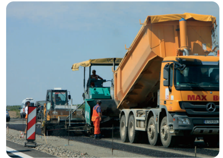
Facility Emergency Repairing
